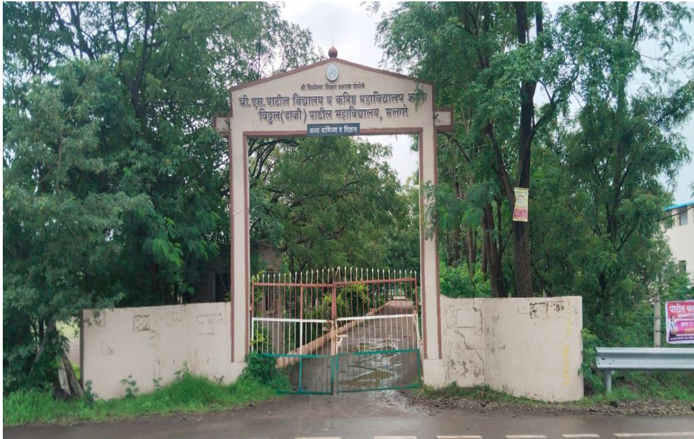
Main Gate ( With Security Guard )
